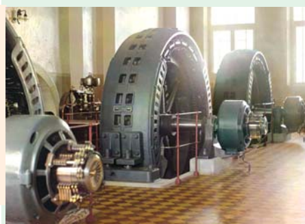
Hydroelectric generators
